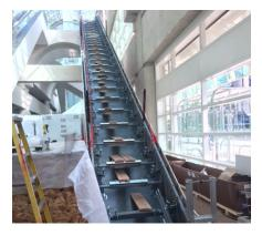
Installation of incline modules is underway on one of the 40-foot units.
